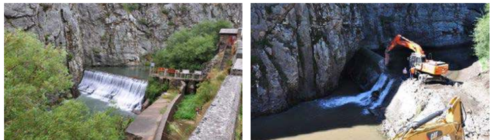
Figure 10: Demolition of La Gotera dam, Spain (© Carlos Marcos Primo, River Duero Basin Authority)
